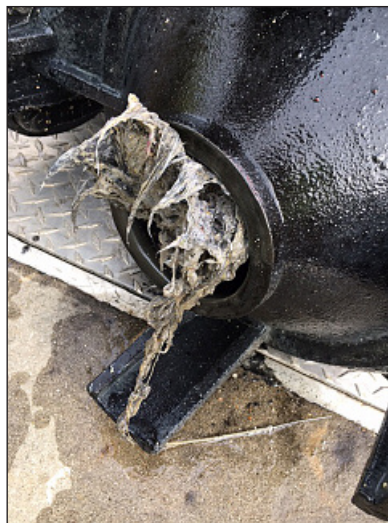
Pictured above: the clogged sewer pump; and a fat berg pulled from the pump.
